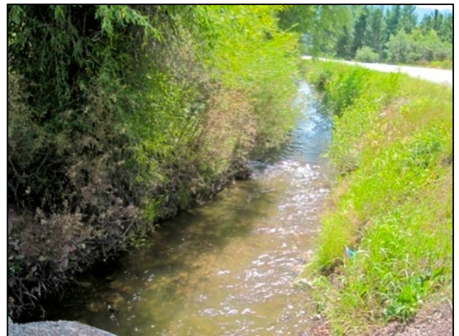
Figure 6. Uncovered earthen canals, like the Salvation Ditch near Aspen, are still considered a reasonably efficient means of conveyance for irrigation water, despite the seepage, evaporation, and phreatophytic growth they permit. (Sharon Clarke)
