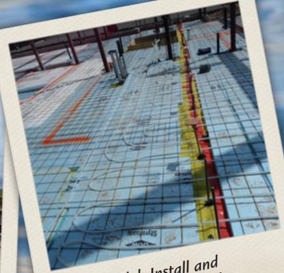
Slab Install and Radiant Heat Piping
