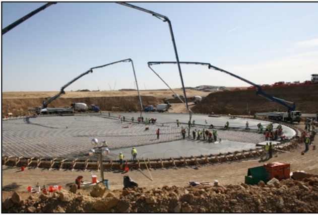
Figure 4. In March of 2009, workers began pouring the foundation for the 10 million gallon Robertsdale Tank, a key component of the Prairie Waters Project. (Aurora Water)
