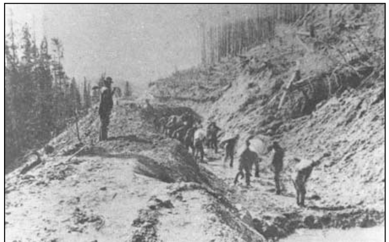
Figure 1. Japanese and Mexican workers dug mile after mile of the Grand Ditch using only picks and shovels (circa 1904). (Fort Collins Museum)
