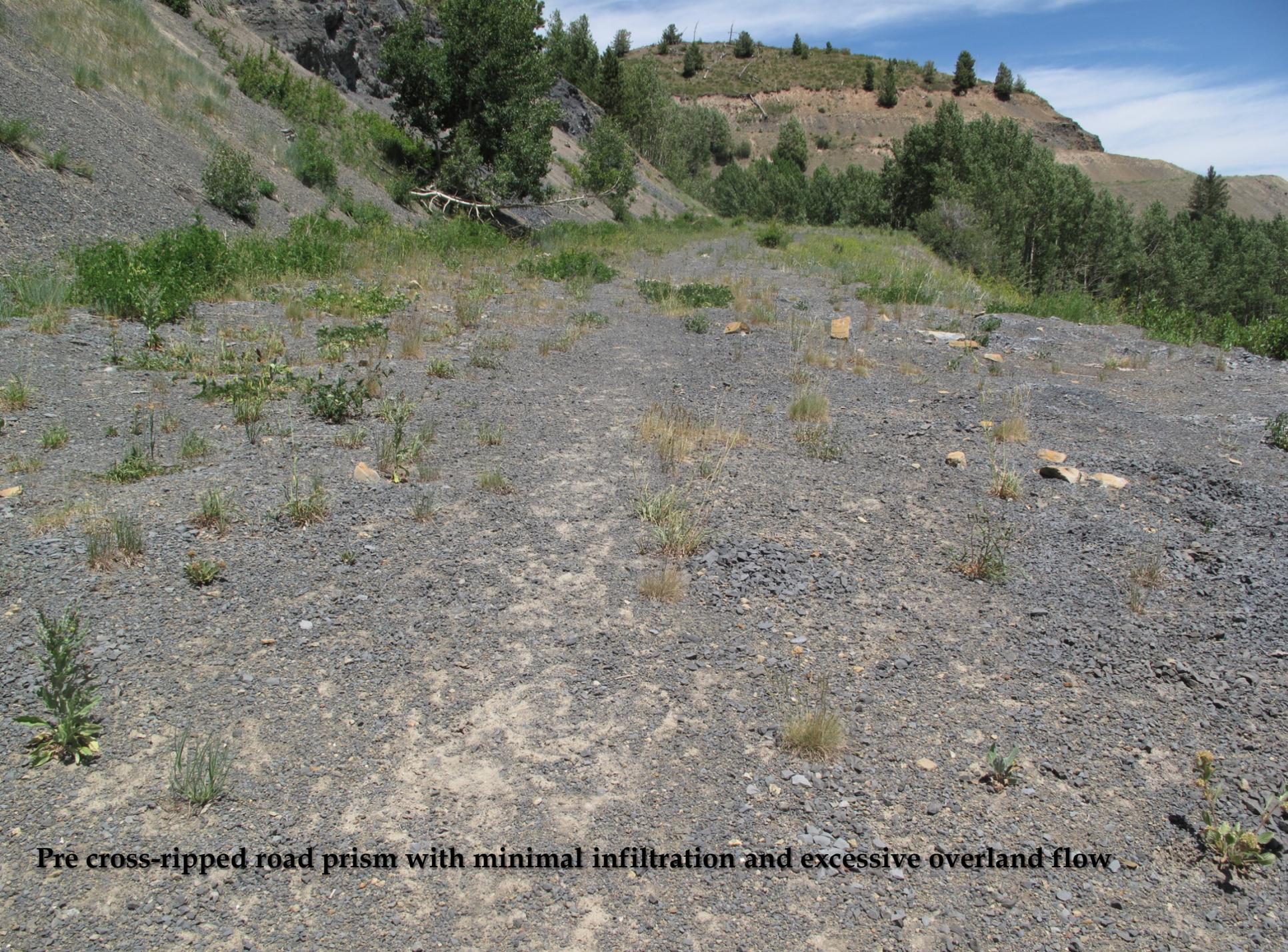
**Pre cross-rippled road prism with minimal infiltration and excessive overland flow**
