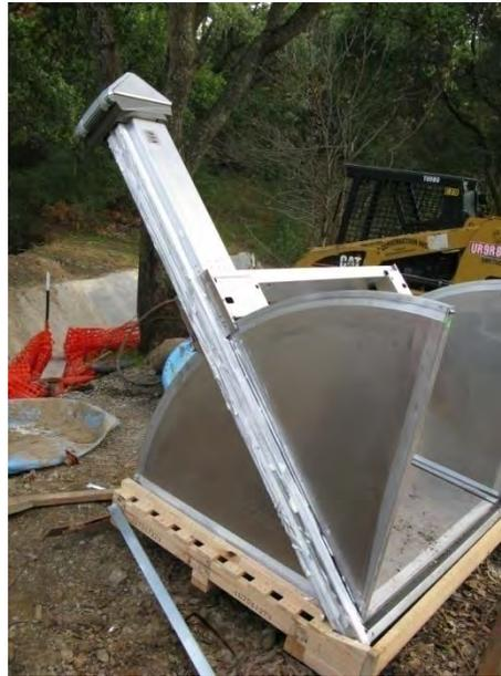
**FlumeGate™ positioned above frame**
