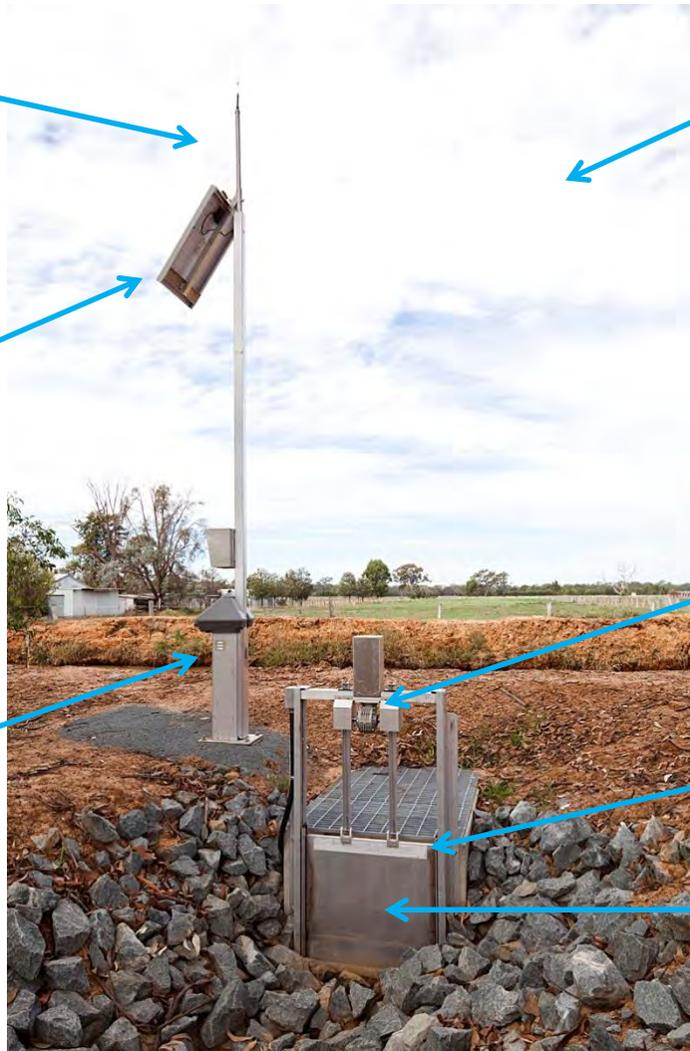
Highly accurate gate control  $\pm 1/16$  of an inch (positive actuation in both directions)
