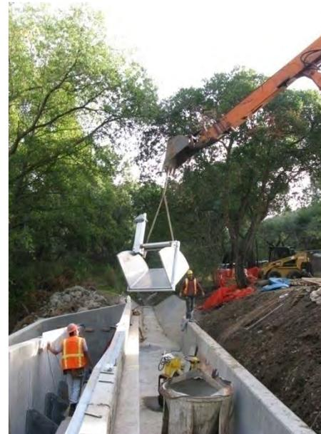
**FlumeGate™ slides into frame – next step is commissioning and then it is ready to pass water**
