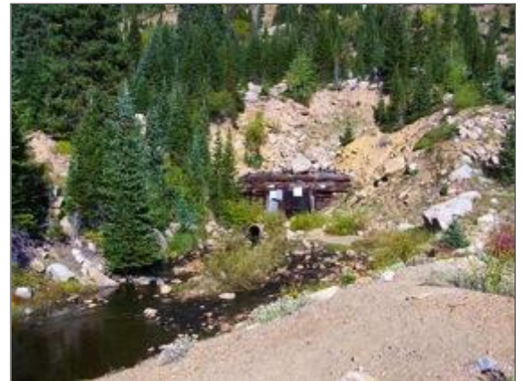
Figure 3. Ivanhoe Tunnel. A pipeline currently comprises the tunnel's diversion capacity, releasing water into Busk Creek, a tributary to Lake Fork Creek.
