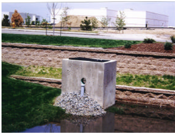
Figure 7: A multi-stage outlet may look like this structure in a detention/water quality pond in Denver. The perforated pipe slowly releases runoff for water quality, the circular opening provides 10-year detention, and the grate on top provides 100-year detention with available freeboard.
