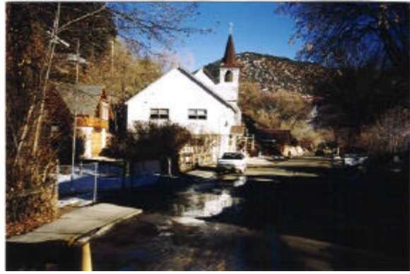
Figure 2: Localized ponding occurs throughout Basalt due to inadequate drainage infrastructure. Storm drains could be constructed to minimize ponding problems, or the area could be regraded.
