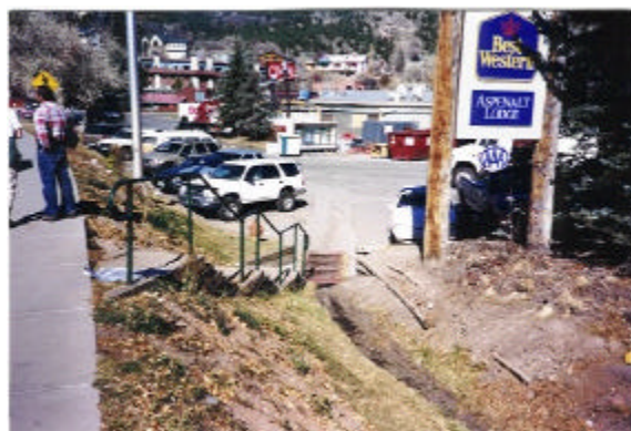
Figure 11: This storm outfall for the Basalt Center Circle is Sample Point 6. Stormwater runoff from the commercial operations within this 6.6-acre basin can introduce pollutants into the Fryingpan River.
