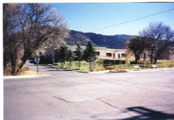
Figure 12: 29 acres are tributary to this inter-section at Cottonwood Drive and Two Rivers Rd. The intersection is prone to local flooding, and a cross pan is needed along with a new culvert.
