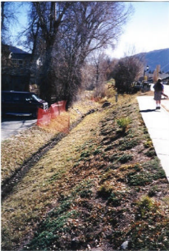
Figure 13: This storm drain outfall for the Basalt Center Circle provides some water quality benefit by disconnecting the impervious surfaces with this grass swale. Regular maintenance is necessary to remove deposited sediment and debris. A pond would provide better treatment.
