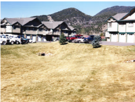
Figure 5: This sedimentation pond in the Elk Run Subdivision creates an opportunity for water quality treatment by constructing a multi stage outlet.
