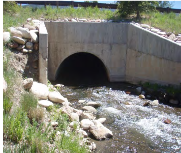
Culvert below roundabout at Brush Creek and Highline Rds
