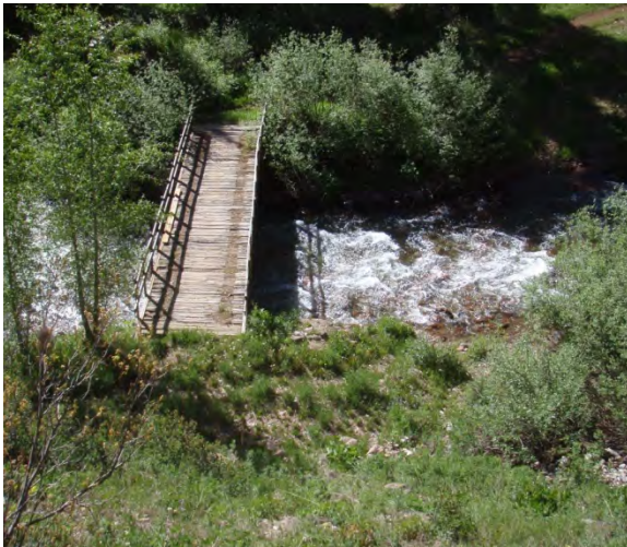
Potential gage site at Footbridge below city diversion structure, access is currently prohibited.
