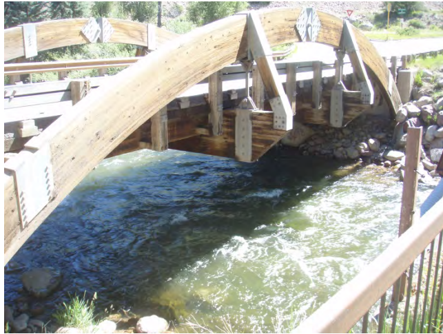
Smith Way Road Bridge and pedestrian bridge
