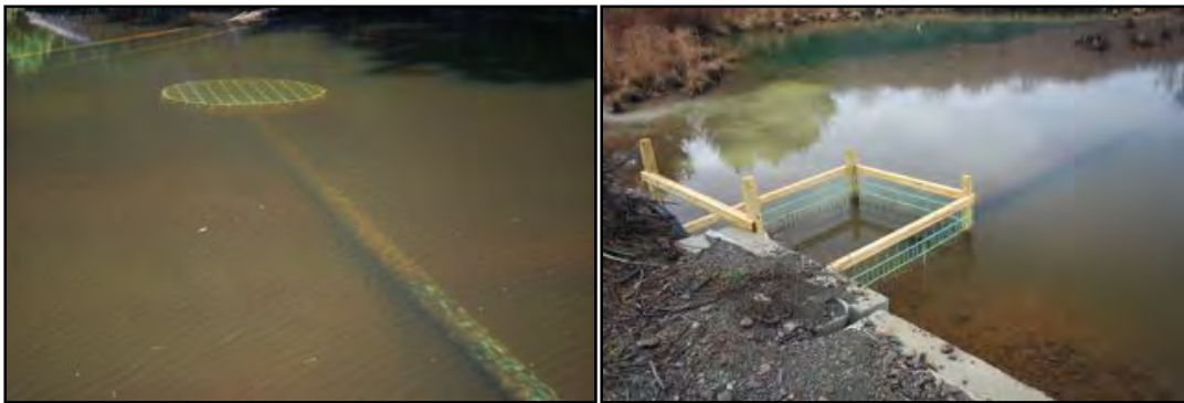
Figure 14. Left photo, Castor Master - A PVC pipe is inserted through a beaver dam extending both upstream and downstream. The upstream end of the pipe in the pond has a grate or the pipe is perforated. The beaver pond will be lowered to the level of the grate or the perforated pipe. Right photo, Beaver Deceiver- A perforated pipe is placed on the upstream side of a culvert and extends into the pond. A fence is constructed at the culvert inlet which the beavers plug, but they cannot plug the perforated pipe that runs into the culvert and extends into the upstream side of the pool (Photo credit: Skip Lisle).
