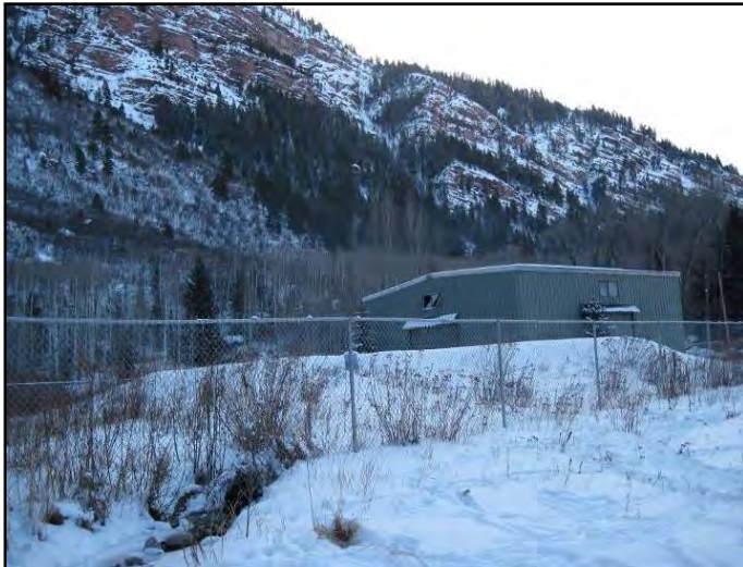
Figure 10. Redstone wastewater treatment plant, January 13, 2011. The Redstone treatment plant recently received a grant to assist with financing the upgrades necessary to remedy the treatment issues which have existed at the facility for several years.
