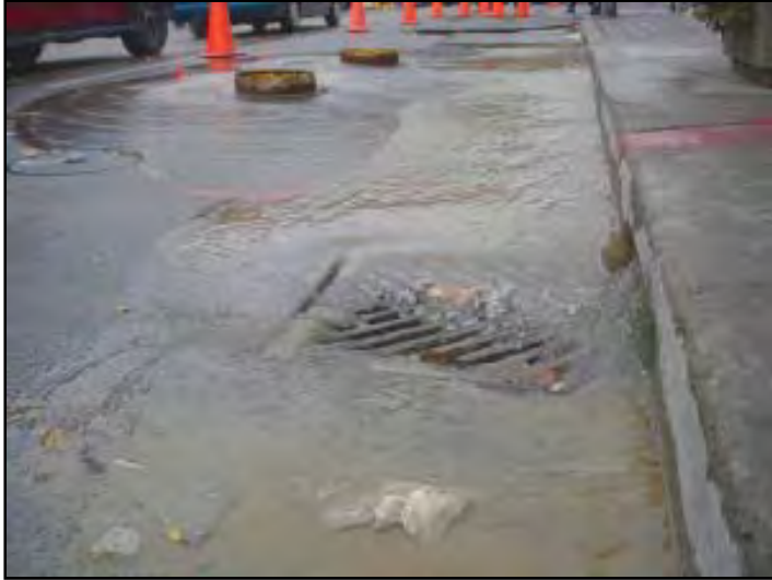
Figure 9. Urban runoff is concentrated in storm drains.
